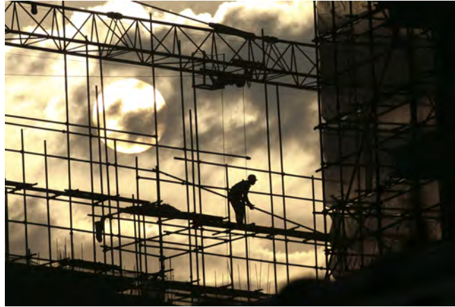
A laborer works on the scaffolding at a construction site in Wuhan, Hubei Province on November 26, 2008. Photo credit: Stringer/REUTERS
